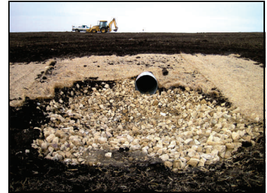
Grade Stabilization Washington Lake Township
